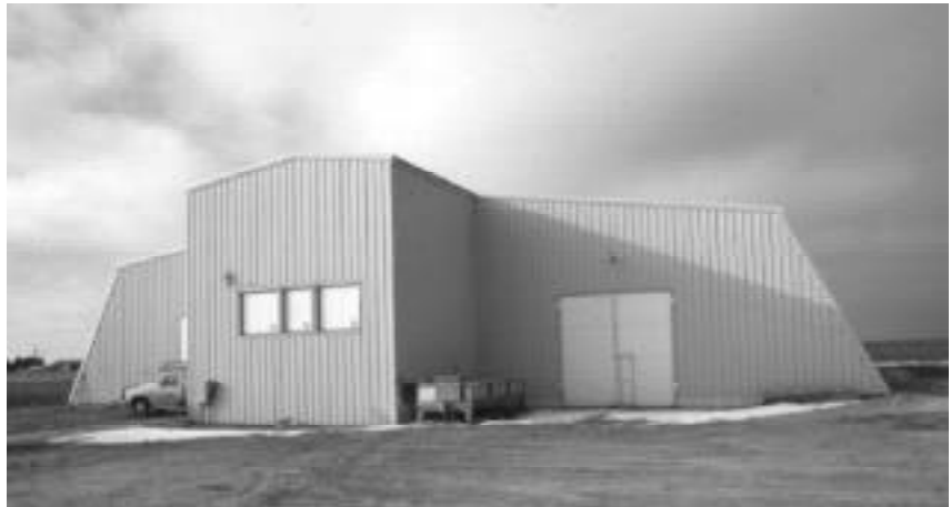
Figure 1. Facility for storing 250,000 cwt of potatoes. This storage has a center plenum for delivery of air into two separate storage bays.
